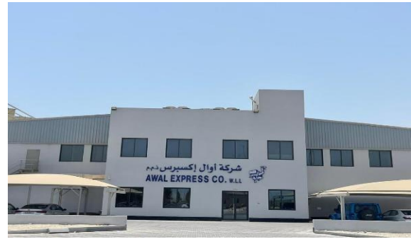
AWAL EXPRESS PROJECT
