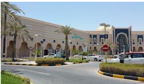
SEEF MALL PROJECT
