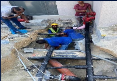
HDPE PIPE WORK IN NEW BAHRAIN INTERNATIONAL AIRPORT
