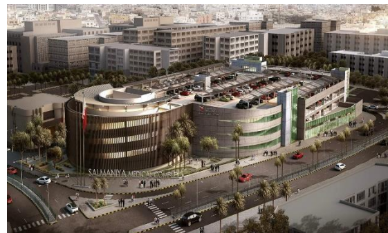
SALMANYA CAR PARK PROJECT
