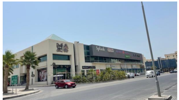
AL HAYAT MALL PROJECT
