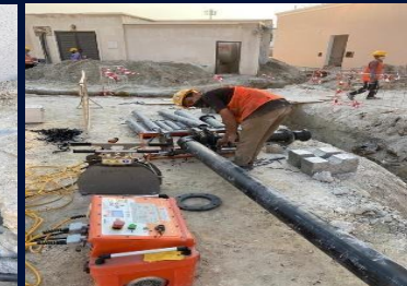
HDPE PIPE WORK IN NEW BAHRAIN INTERNATIONAL AIRPORT
